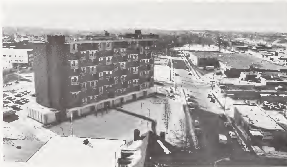
Residential Building (NBS)
